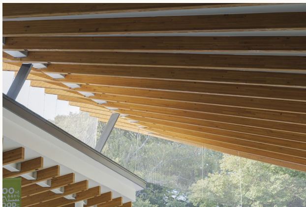
02 架構 — BENEATH THE ROOF
